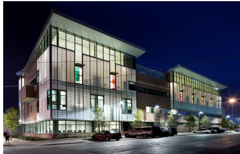
Figura 21: Fachada The Bridge
