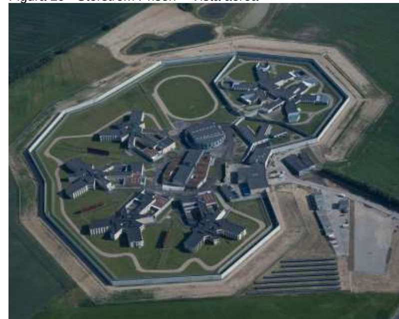
Figura 29 - Storstrom Prison – Vista aérea
