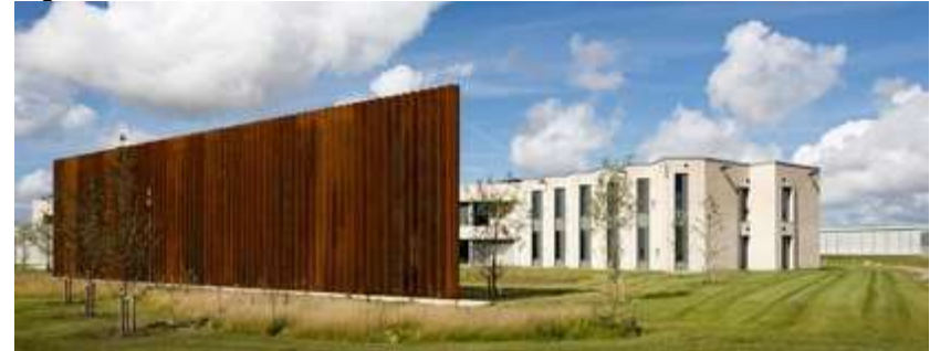
Figura 33 - Storstrom Prison – Fachada externa
