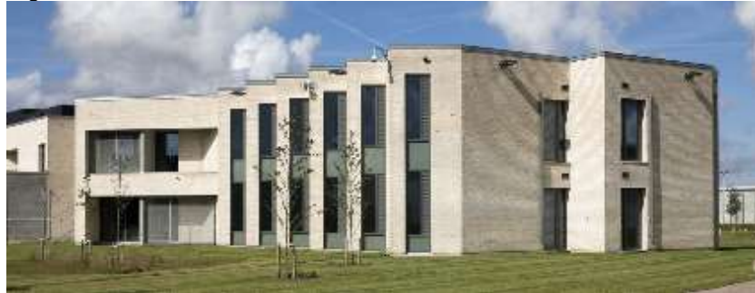
Figura 31 - Storstrom Prison – Fachada externa.
