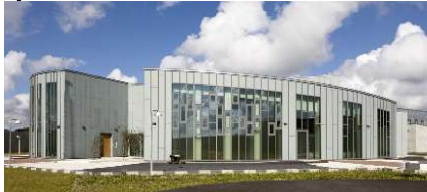
Figura 32 - Storstrom Prison – Fachada externa
