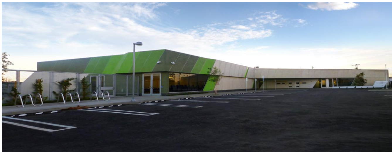
Figura 13. Estacionamento do South Los Angeles Animal Care Center and Community Center.
