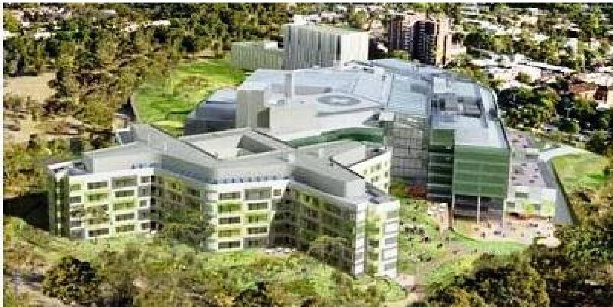
Figura 23 - Fachada principal Royal Children's Hospital Fonte: Mariart Design Studio, 2020.
