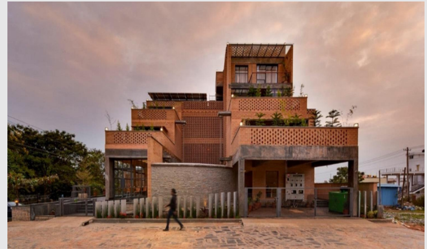
Figura 17: Fachada Sunyata Eco Hotel
